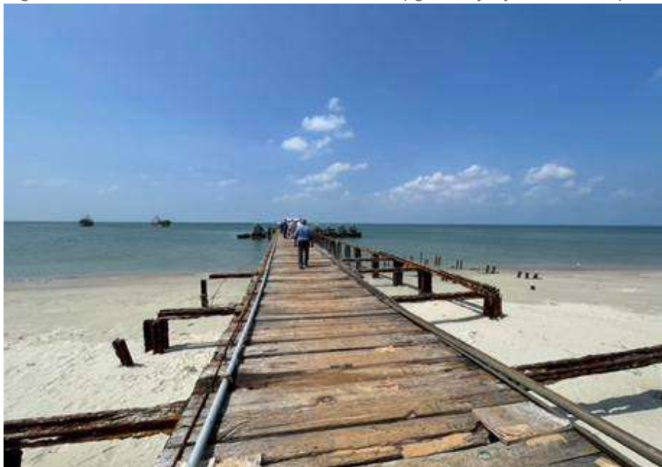
Figure 79 Photo from the site visit to the to-be-upgraded jetty near Thalvupadhu Naval Base
