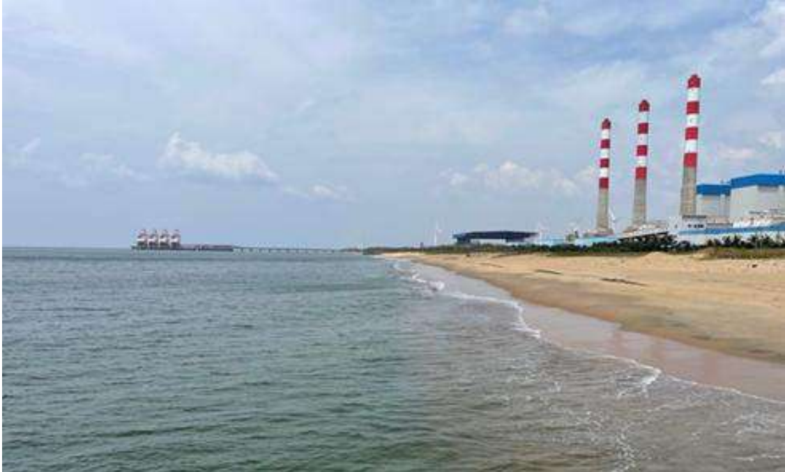
Figure 85 Photo taken on the to-be-upgraded jetty near Norochcholai Power Plant, overlooking the Lakvajiya coal jetty
